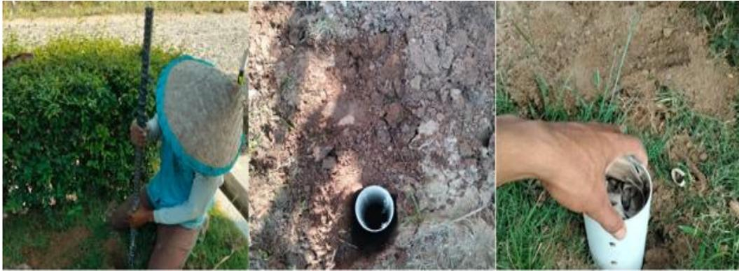
**Gambar 5 Proses instalasi biopori**
